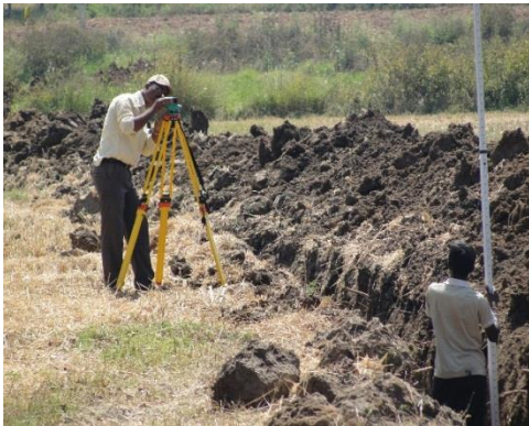
A view of survey before installation of sub surface drainage
